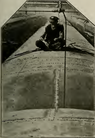
WELDING ROOF JOINT TIGHT ON A STEEL PASSENGER CAR.
